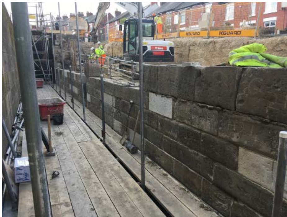
Lock 15 wall reconstruction
