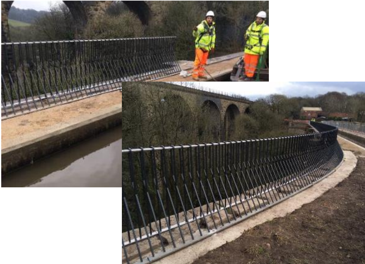
Marple Aqueduct safety fencing
