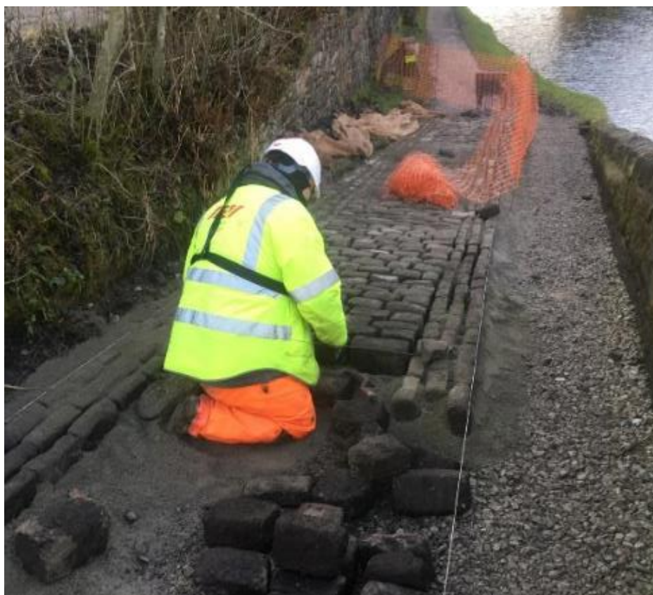
Towpath ramp reconstruction using stone setts
