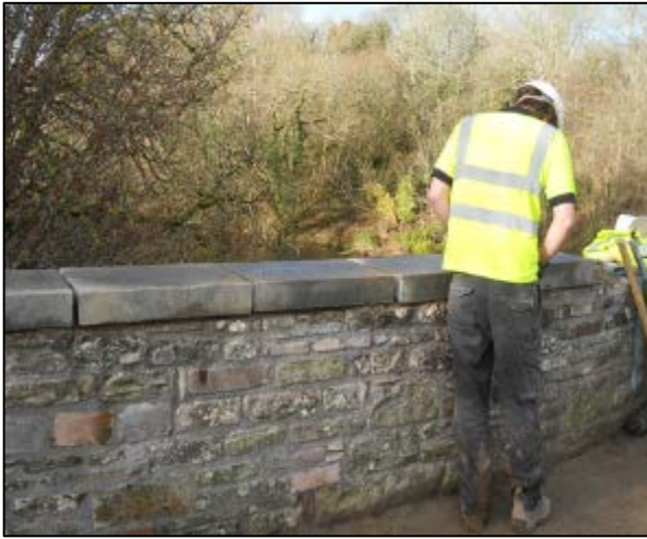
Brynich Aqueduct, M&B Canal
